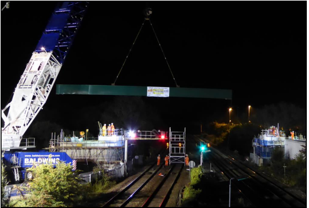
above: In the early hours of Sunday 3 rd September, the first girder of the new bridge across the Midland main line is lowered into position.
